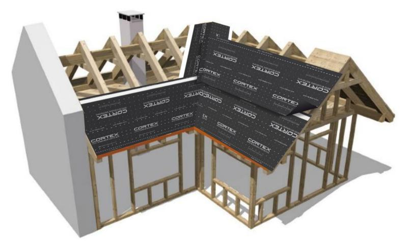
Install the next piece of membrane with the bottom edge lining up with the 100mm overlap line and overlapping the verge. Install the membrane over any valleys and onto the adjacent pitch. Tack the membrane in place.
