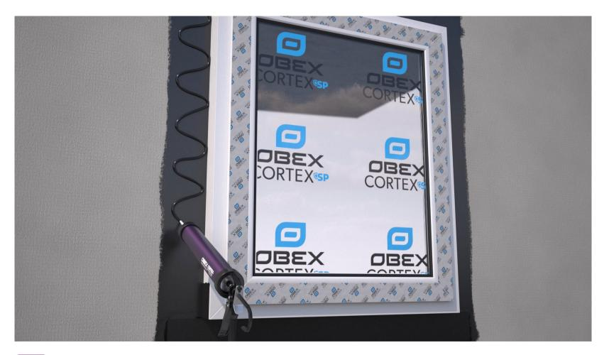
Apply OBEX CORTEX 0769 Paste Adhesive to the sides of the frame and substrate.
