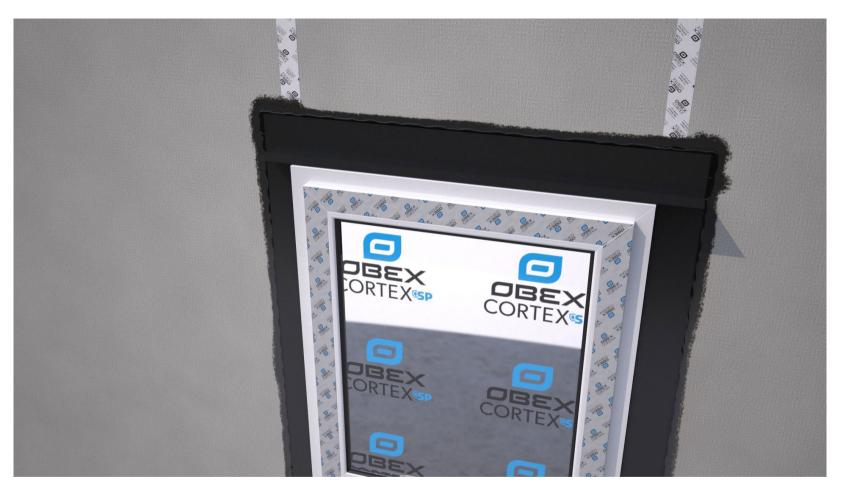
Bond the EPDM Membrane to the frame first, and then bond back to the substrate. Ensure the membrane is applied flat, without creases, and tension free.
