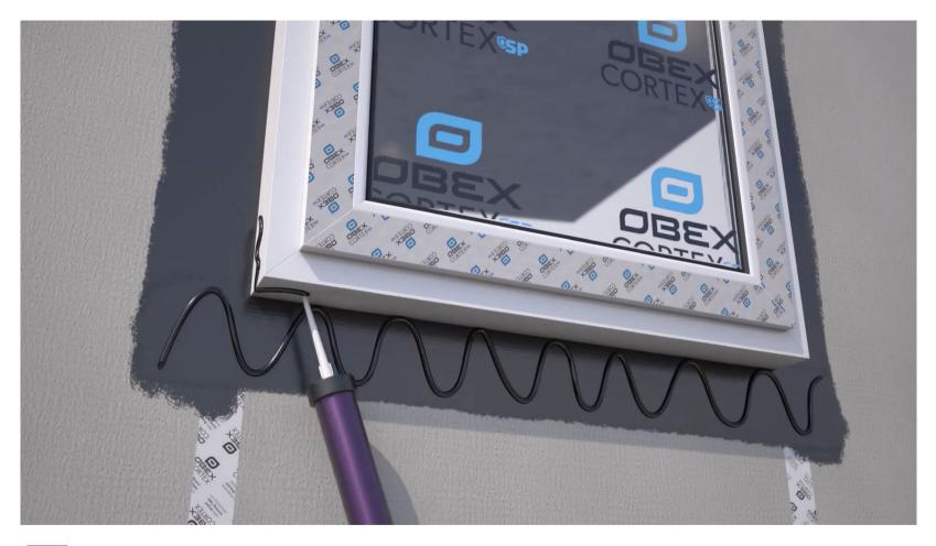
Apply OBEX CORTEX 0769 Paste adhesive to the frame and substrate surface using a paste adhesive gun.
