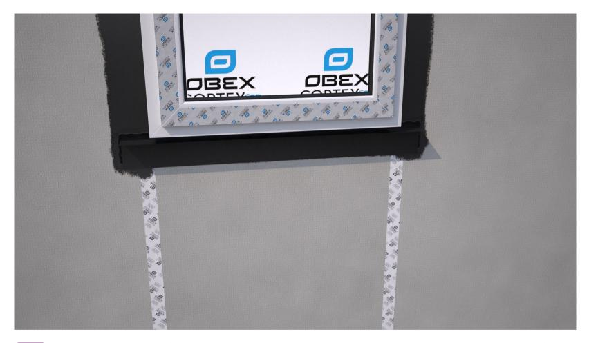
Bond the EPDM Membrane to the frame first, and then bond back to the substrate. Ensure the membrane is applied flat, without creases, and tension free. It is mandatory that the cill membrane is installed first.
