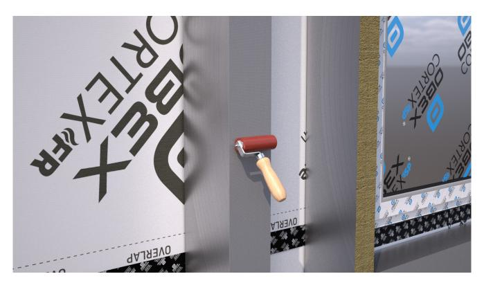
Firmly roll over the membrane with a rubber roller, ensuring to cover the full width of the cavity barrier below.
