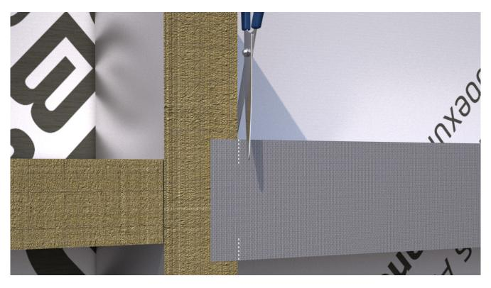
Cut the membrane flush with the vertical barrier, so that it can be folded over the horizontal barrier.
