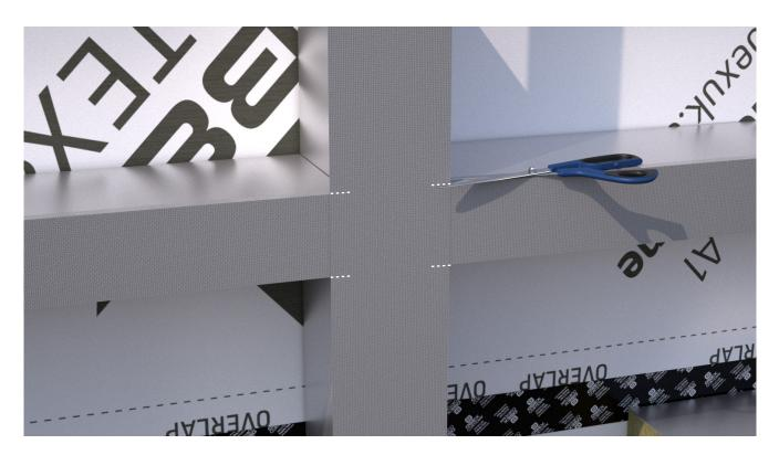
For vertical sections, repeat steps 2-5. When there is a joint between a vertical and horizontal barrier, cut the membrane flush with the horizontal, so that the membrane can be folded over the vertical barrier.
