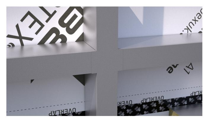
Fold the membrane over and bond onto the vertical cavity barrier's side faces.
