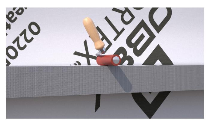
Firmly roll over the membrane to ensure a good bond strenght from the adhesive on the rear of the membrane.
