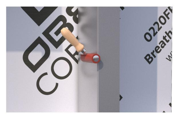
Ensure to roll over the sides of the membrane with firm pressure to achieve a good bond strength.
