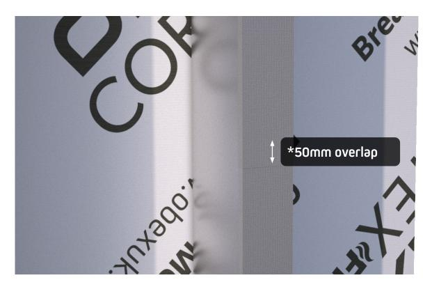
With a new roll of membrane, overlap the lower membrane by at least 50mm, and install as per previous steps.
