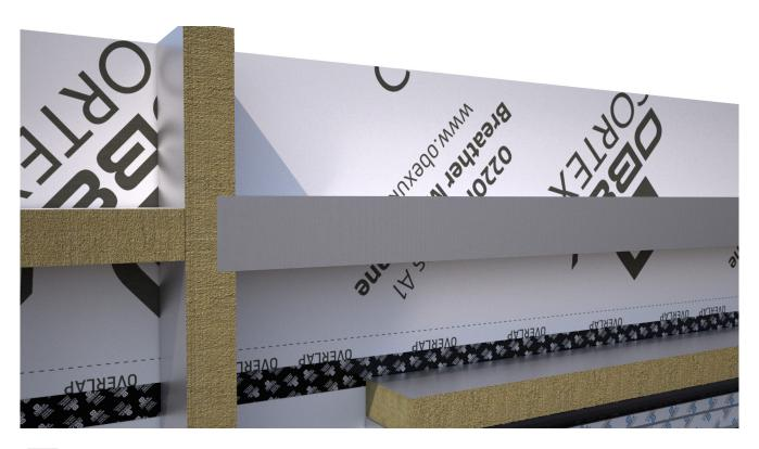
Flip the membrane over and line it up with the horizontal cavity barrier. Ensure there is a 25mm overhang on either side of the barrier, and that it overhangs the vertical barrier by 50mm.
