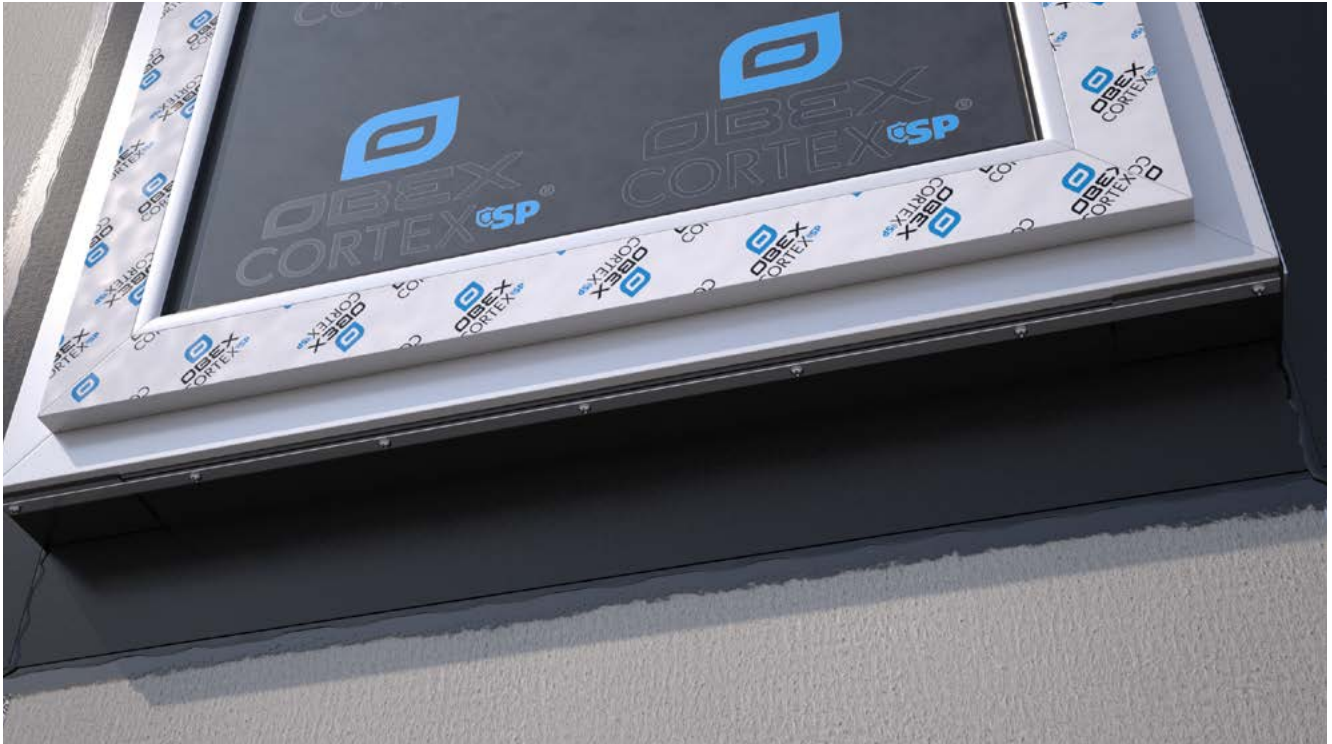
Completed termination bar installation at the base of the window.
