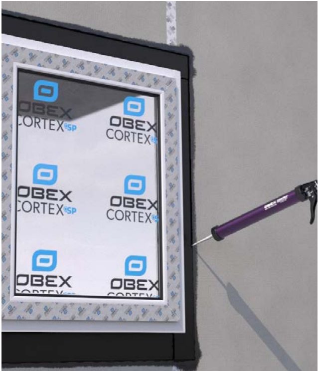
Apply a bead of OBEX CORTEX 0210FR Paste Adhesive around the perimeter and over any joints/overlaps.
