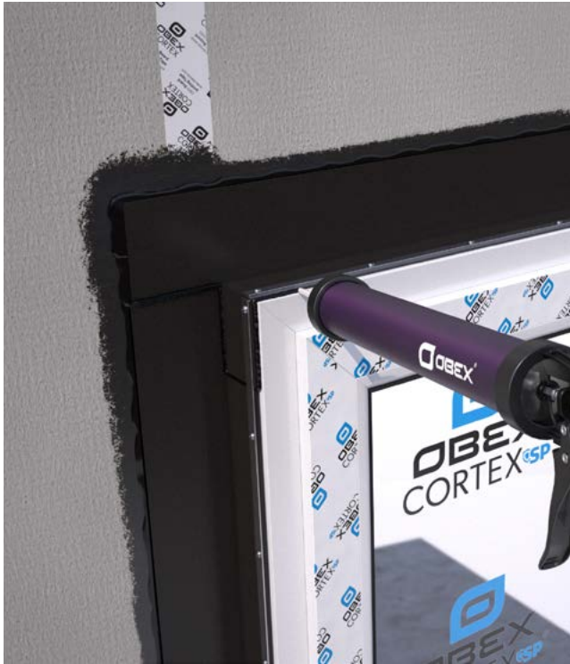
Apply a bead of OBEX CORTEX 0210FR Paste Adhesive around the perimeter and over any joints/overlaps.
