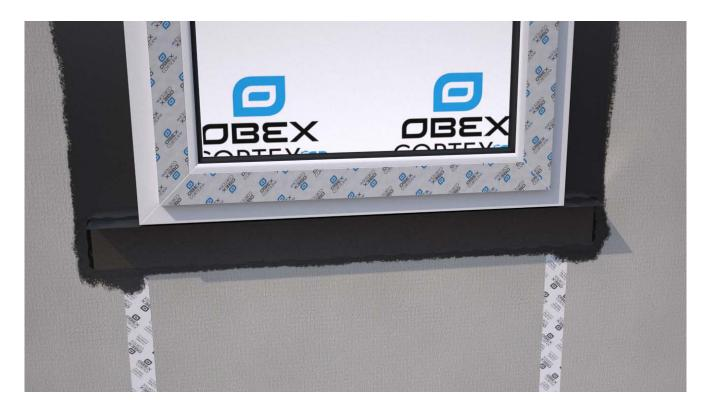
Bond the O200FR Membrane to the frame first, and then bond back to the substrate. Ensure the membrane is applied flat, without creases, and tension free. It is mandatory that the cill membrane is installed first. Important: Ensure membrane is with the silver face to the substrate and the black face exposed.
