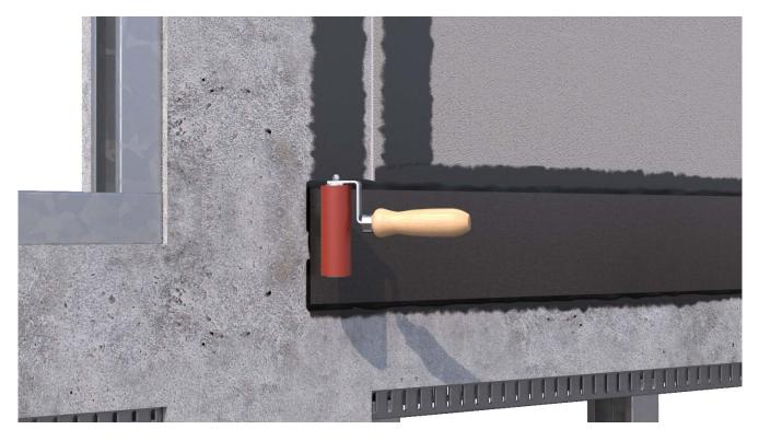
Firmly roll the ISM with a roller to ensure maximum bond strength is achieved.
