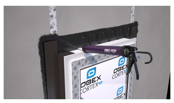
Apply OBEX CORTEX 0210FR Paste Adhesive to the head of the frame and substrate.
