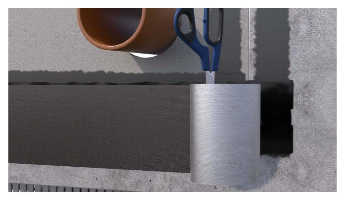
Unroll OBEX CORTEX 0200FR Interface Sealing Membrane and cut to required length using membrane shears.
