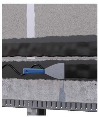
Apply OBEX CORTEX 0210FR Class A2 Paste Adhesive to the sheathing board and slab edge (100mm min width). Spread the paste using a scraper ensuring an even spread at 1-2mm thickness.
