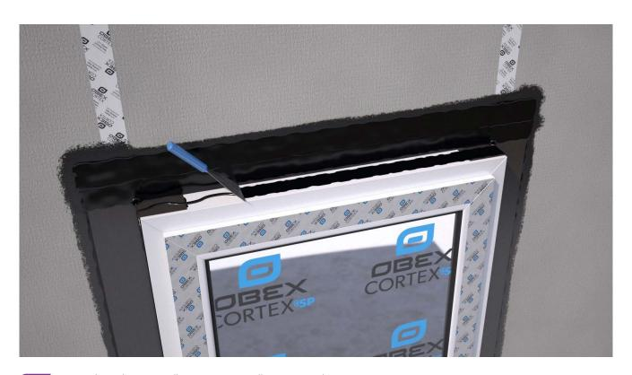
Spread out the paste adhesive using an adhesive spreader.
