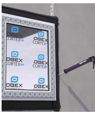
Apply a bead of OBEX CORTEX 0210FR Paste Adhesive around the perimeter and over any joints/overlaps.
