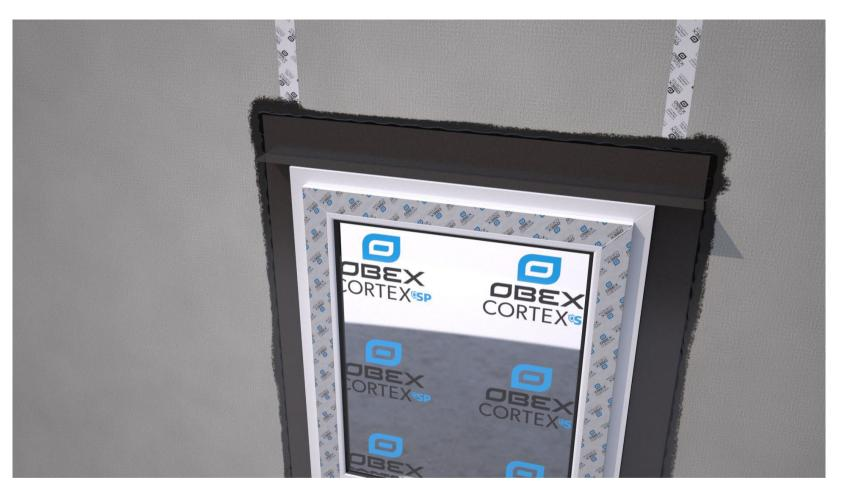
Bond the 0200FR Membrane to the frame first, and then bond back to the substrate. Ensure the membrane is applied flat, without creases, and tension free.
