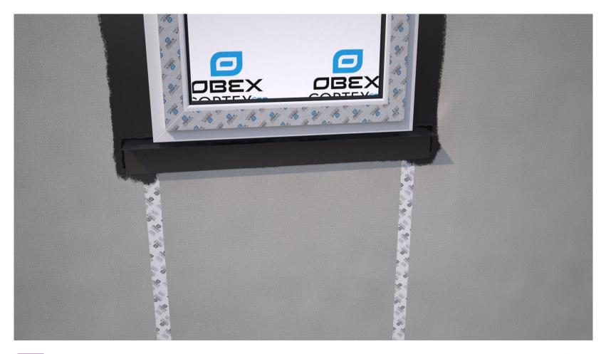
Bond the 0200FR Membrane to the frame first, and then bond back to the substrate. Ensure the membrane is applied flat, without creases, and tension free. It is mandatory that the cill membrane is installed first.
