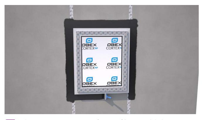
Apply OBEX CORTEX 0787FR Primer to porous surfaces. Ensure a full coverage over the bonding area. Porous surfaces include cement board, calcium silicate board, concrete etc.
