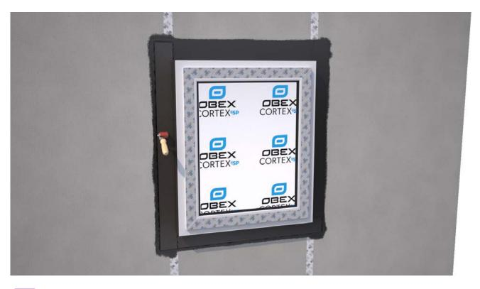
Roll firmly with a seam roller to ensure maximum bond strength to the frame and the substrate.
