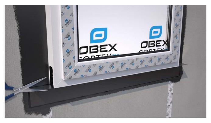
Create an incision as shown by the scissors. Fold and bond the membrane up the frame, ensuring it's applied flat and without creases.
