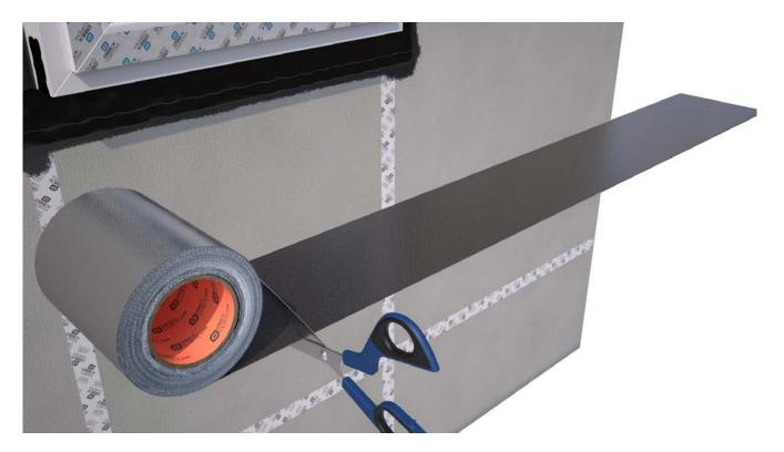
Cut the 0200FR Membrane to length. Ensure the length of membrane extends at least 100mm past each side of the window.
