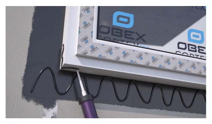
Apply OBEX CORTEX 0210FR Class A2 Paste adhesive to the frame and substrate surface using a paste adhesive gun.
