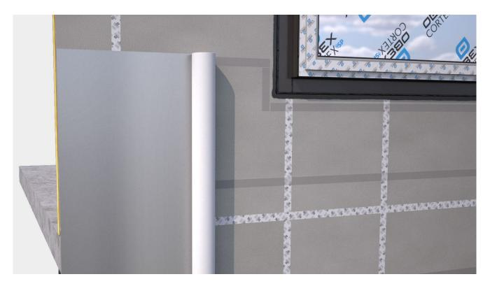
You're now ready to apply the breather membrane. Place the roll into position to cover the strips of double-sided tape and start rolling the membrane over the tape. The membrane should be installed with the silver side facing out from the building.
