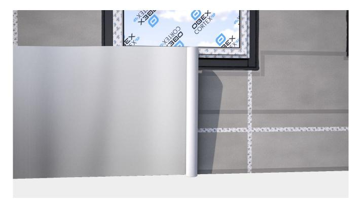
Where possible, the membrane should be continuous so any window/door openings or penetrations should be cut out during application, or it can be applied over the top and cut out afterwards.
