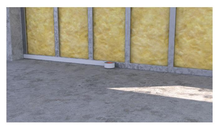
Start by applying the OBEX CORTEX 0824FR Double-Sided Tape to the base track. Consider where fixings may penetrate the vapour control layer and ensure that double-sided tape is present at these locations. Do not apply d/s tape to the head track - this is to allow for expansion/contraction.
