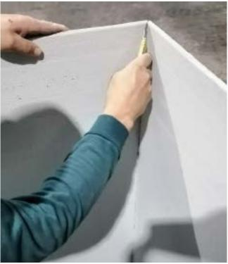
Once the desired dimensions have been marked on the board, using a suitable knife, score the board with a single firm cut on one side ensuring the mesh has been cut. Firmly bend and snap the board along the initial cut, and then cut the mesh on the reverse side.
