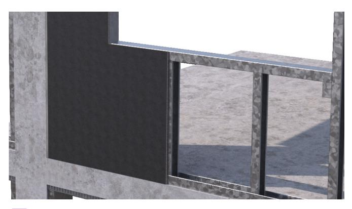
Offer up the board into position, ensuring the edges of the board are just shy of the centre line of the framing member to leave the recommended 3-5mm gap.
