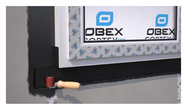
Roll firmly with a seam roller to ensure maximum bond strength to the frame and the substrate.
