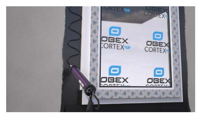
Apply OBEX CORTEX 0771FR Paste Adhesive to the sides of the frame and substrate.
