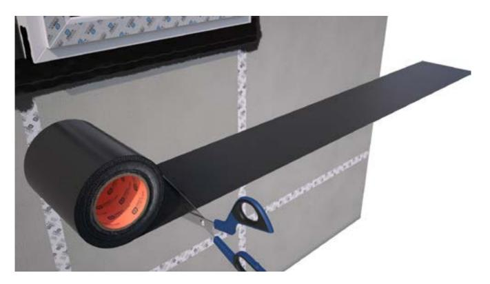
Cut the 0500FR Membrane to length. Ensure the length of membrane extends at least 100mm past each side of the window.
