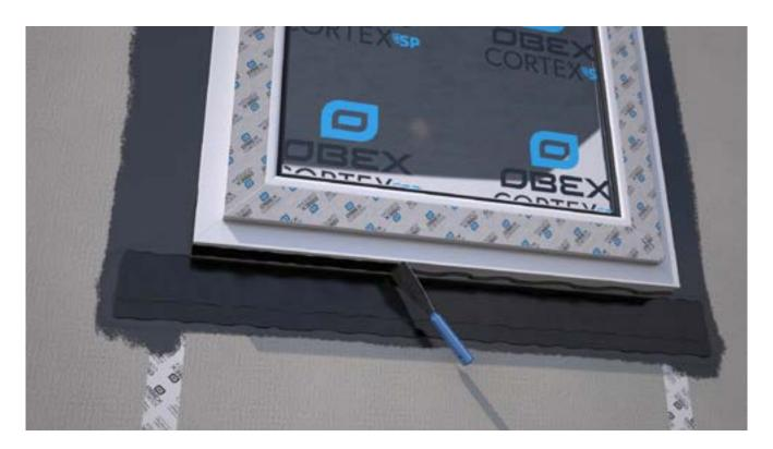
Spread out the 0771FR paste using an adhesive spreader.
