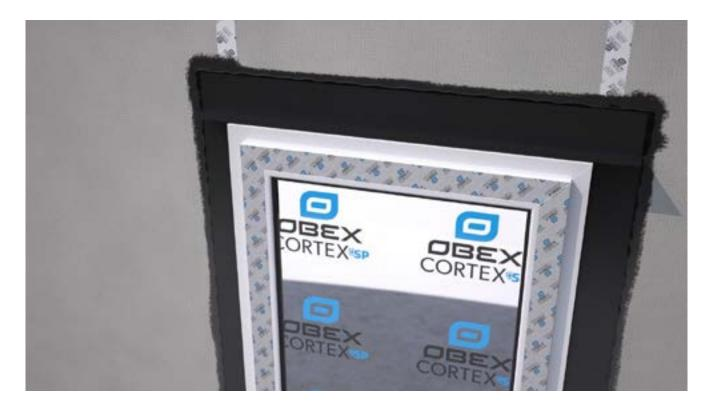
Bond the 0500FR Membrane to the frame first, and then bond back to the substrate. Ensure the membrane is applied flat, without creases, and tension free.
