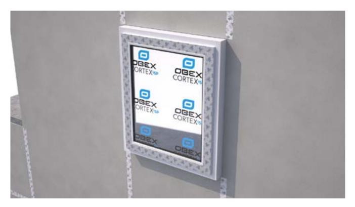
Ensure the window surround is complete and ready to receive the ISM. Mark up the substrate to ensure the correct bond widths are achieved. The required bond widths are; 100mm onto porous surfaces (concrete etc) and a minimum of 20-30mm onto non-porous surfaces.
