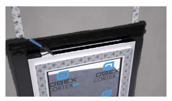
Spread out the paste adhesive using an adhesive spreader.
