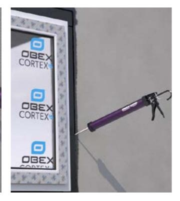
Apply a bead of OBEX CORTEX 0771FR Paste Adhesive around the perimeter and over any joints/overlaps.
