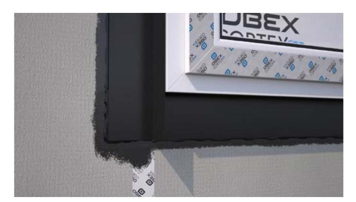
Bond the O500FR Membrane to the frame first, and then bond back to the substrate. Ensure the membrane is applied flat, without creases, and tension free.
