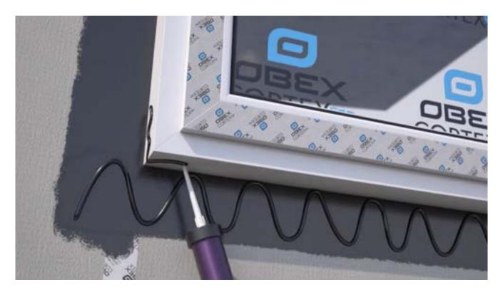
Apply OBEX CORTEX 0771FR Class B Paste adhesive to the frame and substrate surface using a paste adhesive gun.
