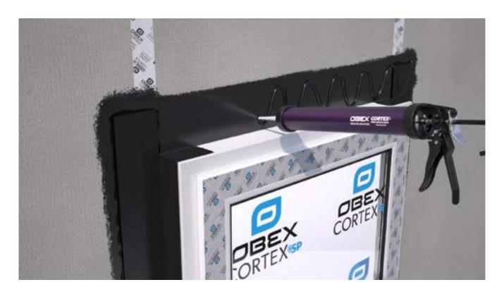
Apply OBEX CORTEX 0771FR Paste Adhesive to the head of the frame and substrate.
