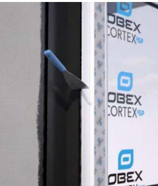
Tool off the paste adhesive using an adhesive spreader and ensure there are no open edges.
