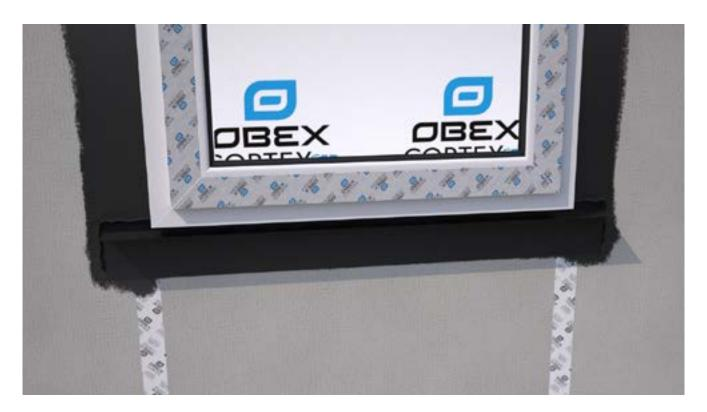
Bond the 0500FR Membrane to the frame first, and then bond back to the substrate. Ensure the membrane is applied flat, without creases, and tension free. It is mandatory that the cill membrane is installed first.
