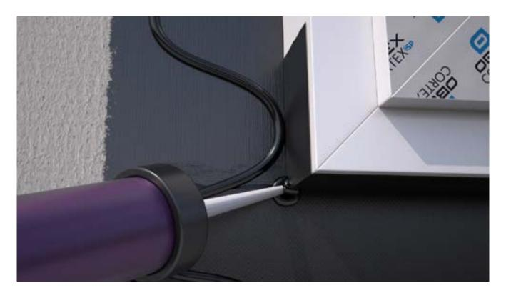
IMPORTANT: Apply a small bead of paste adhesive at corner location. This is to ensure the corners are adequately sealed.
