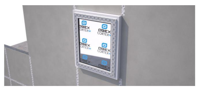
Ensure the window surround is complete and ready to receive the ISM. Mark up the substrate to ensure the correct bond widths are achieved. The required bond widths are; 100mm onto porous surfaces (concrete etc) and a minimum of 20-30mm onto non-porous surfaces.
