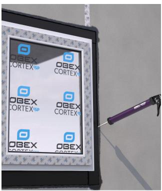
Apply a bead of OBEX CORTEX 0771FR Paste Adhesive around the perimeter and over any joints/overlaps.
