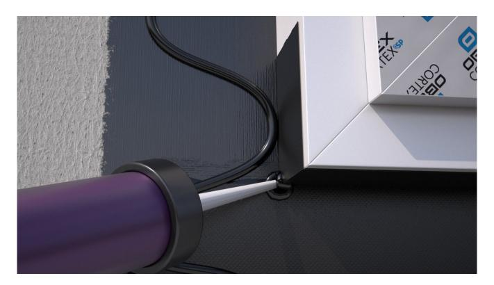
${\tt IMPORTANT: Apply \ a \ small \ bead \ of \ paste \ adhesive \ at \ corner \ location. \ This \ is \ to \ ensure \ the \ corners \ are}$ adequately sealed.
