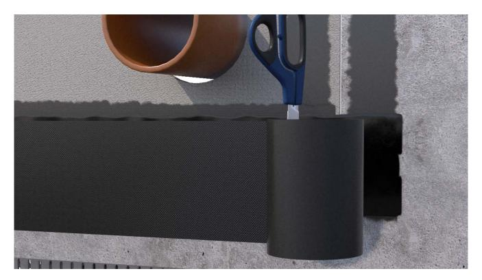
Unroll OBEX CORTEX 0500FR Interface Sealing Membrane and cut to required length using membrane shears.
