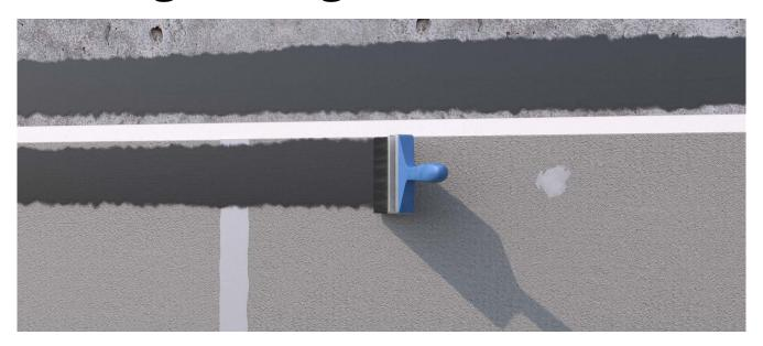
Apply OBEX CORTEX 0787FR Non-Flammable Surface Primer to the concrete slab edge and sheathing board in excess of 100mm width. Allow to flash-off (usually 10 minutes in recommended application temperatures).
