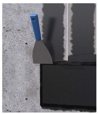
Apply a cap-off bead of paste to the edges of the membrane and spread to ensure a smooth finish.
