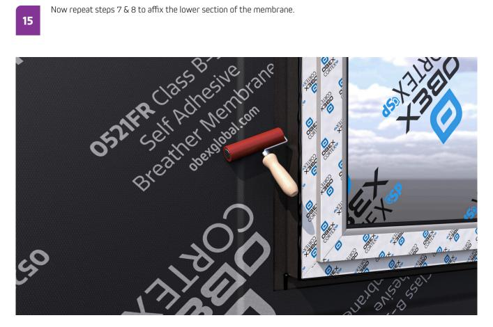
Use the roller to ensure that the edge of the membrane is bonded firmly onto the ISM around the window.
