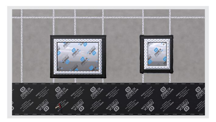
Remove the release liner and affix the lower half of the membrane, using the roller to ensure a good bond.
