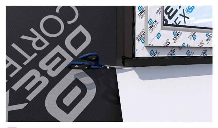
Once the end of the section is reached, remove the window cutout, allowing a 100mm overlap onto the ISM.
