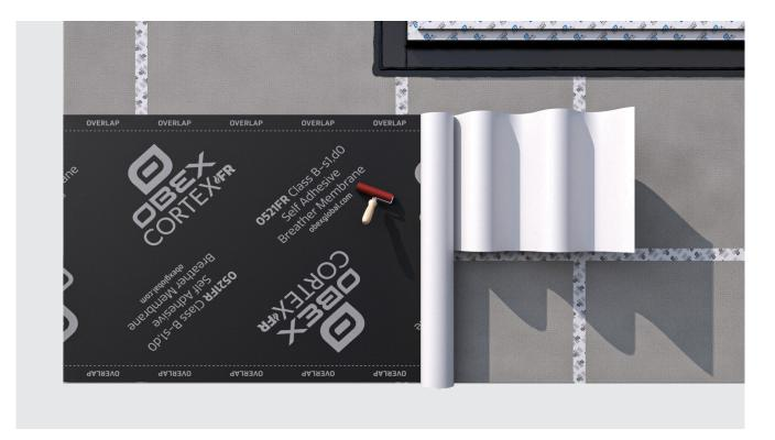
Continue to remove the top release liner, whilst simultaneously applying the membrane to the substrate. Use the roller to ensure it is firmly adhered.
