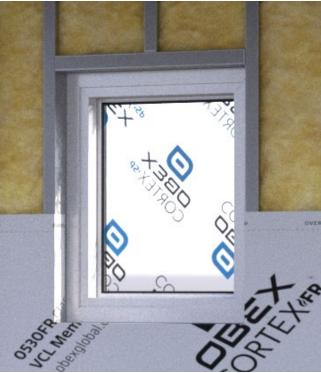
Where possible, the membrane should be continuous so any penetrations should be cut out during application, or it can be applied over the top and cut out afterwards.
