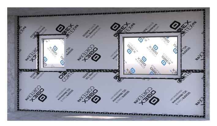
Seal off all edges and joins with OBEX CORTEX 0823FR UV Façade Tape, including where the membrane junctions with other VCLs or the head/floor concrete slab.
