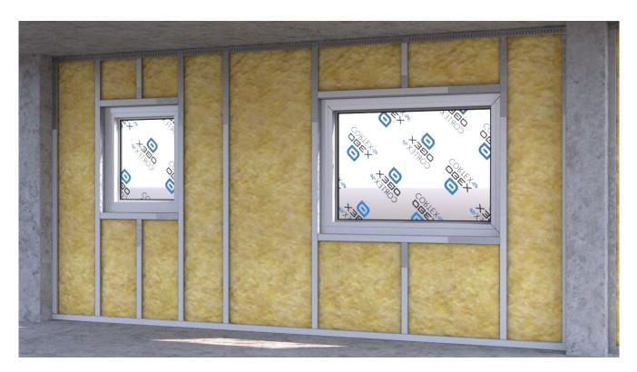
Apply OBEX CORTEX 0824FR Double-Sided Tape to the vertical studs, considering where fixings may penetrate the vapour control layer and ensure that double-sided tape is present at these locations. Do not apply d/s tape to the head track - this is to allow for expansion/contraction.
