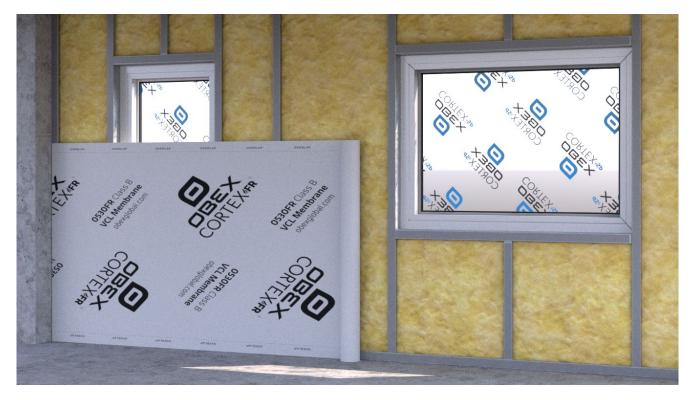
Apply the vapour control layer over the double-sided tape in horizontal strips starting from the base. It is recommended that the next layer should overlap the previous layer by 50mm. The membrane MUST be installed with the printed side visible to the installer.
