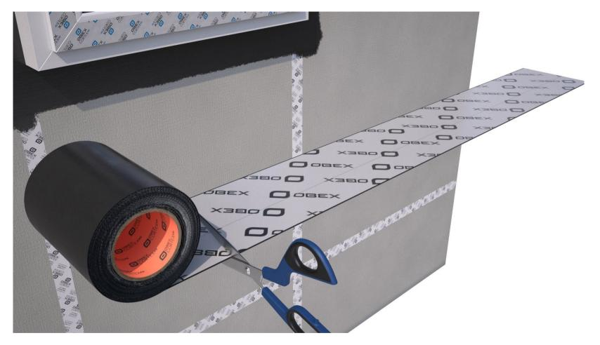
Measure the length of the section and cut the membrane to the correct length. Remember to allow approx. 100mm overlap past the corners of the glazing unit.
