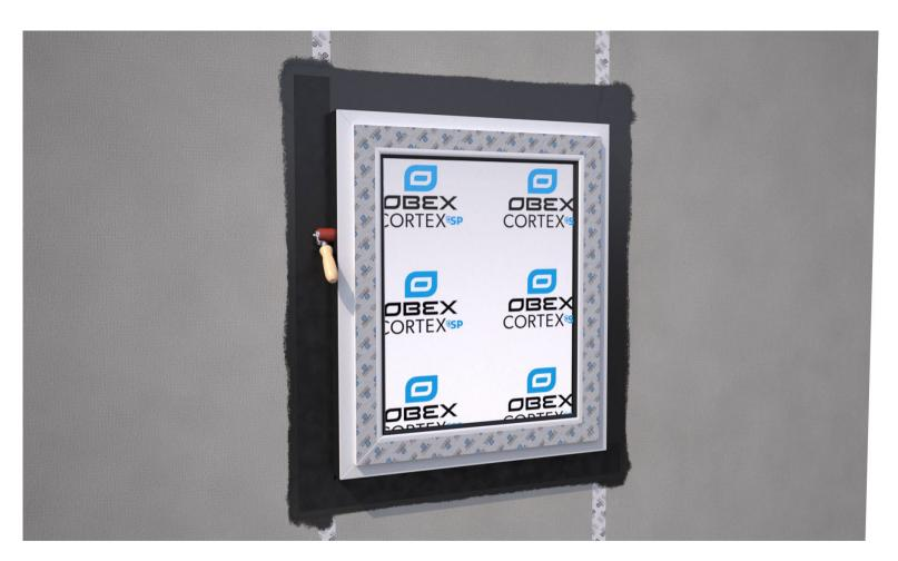
Remove the release liner from the second half of the membrane and bond in place. Ensure all surfaces are firmly rolled for maximum bond strength.
