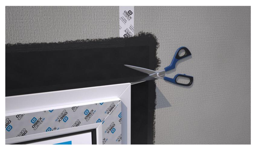
Cut and fold the corner laps into position.
