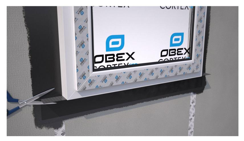
Bond the membrane in position starting at the window frame. Once positioned and bonded, the corner laps can be cut and folded into position.
