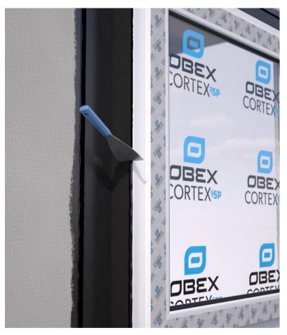
Tool-off the bead of adhesive with a spreader to ensure all edges/joints/overlaps are fully sealed.
