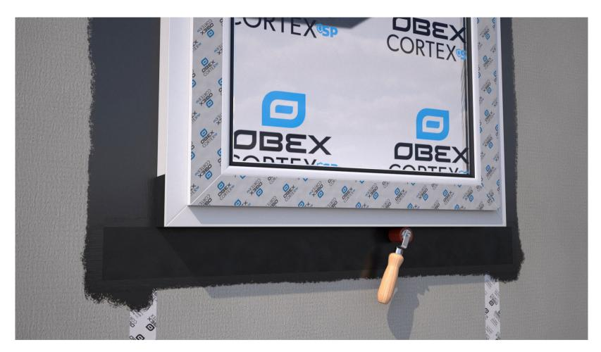
Ensure all surfaces are firmly rolled to ensure maximum bond strength is achieved.
