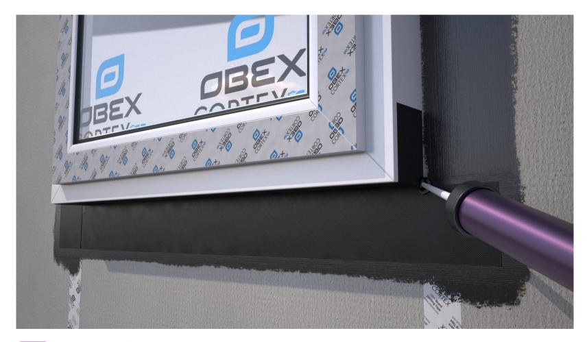
Ensure a small amount of OBEX CORTEX 0771FR Class B Paste Adhesive is applied in the corner areas as shown.
