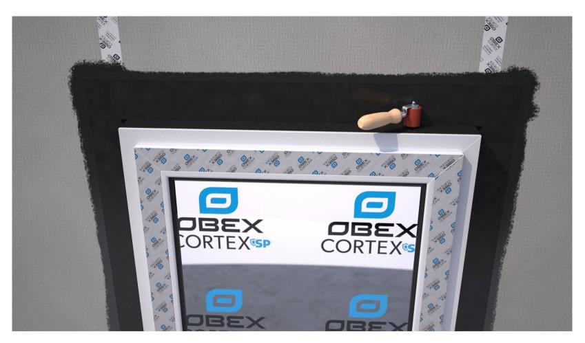
Ensure all membrane surfaces are firmly rolled with a roller for maximum adhesion levels.
