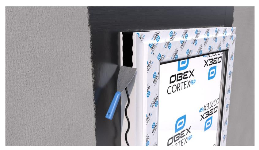
**For Profiled / Rough Windows:** Spread out the 0771FR paste using an adhesive spreader. **For Flat / Smooth Surface Windows: Move onto the next step**
