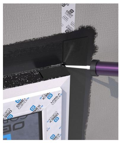
IMPORTANT: Apply a small bead of paste adhesive at corner location. This is to ensure the corners are adequately sealed.
