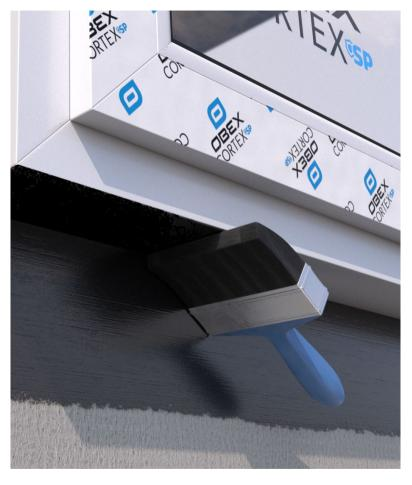
For Profiled / Rough Windows: Apply OBEX CORTEX 0771FR Class B Paste adhesive to the frame using a paste adhesive gun. For Flat / Smooth Surface Windows: Apply OBEX CORTEX 0778FR Class B Contact adhesive to the frame and substrate surface using a brush.
