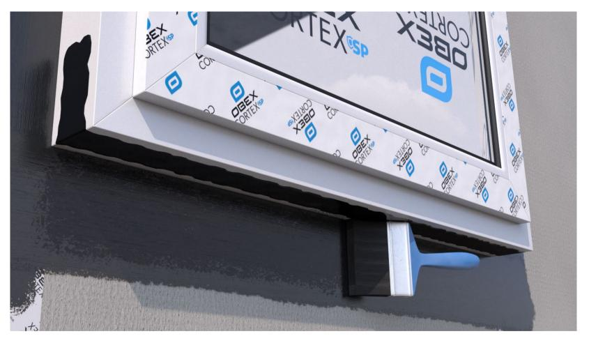
Apply the OBEX CORTEX 0778FR Contact Adhesive onto the substrate using a brush or roller. Ensure a full surface coverage. Leave for 10 minutes to flash off.
