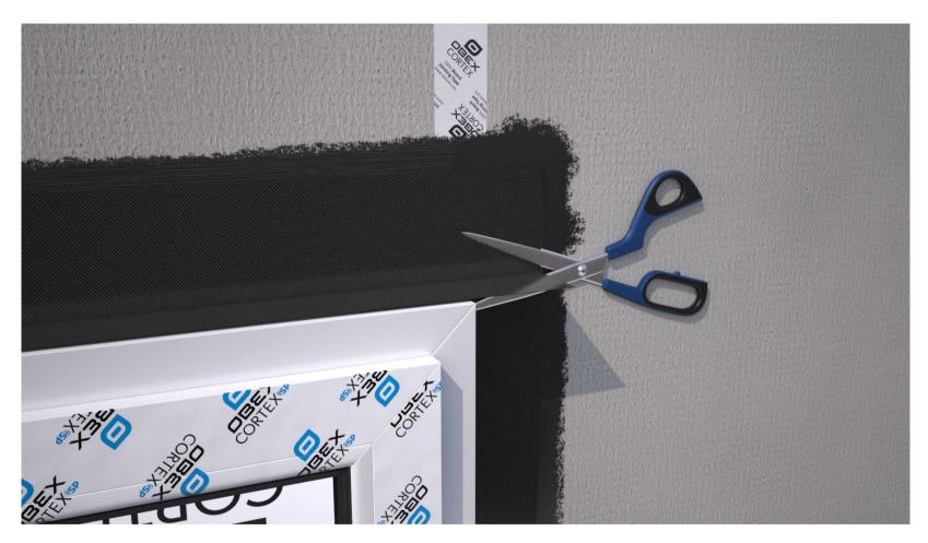
Create an incision as shown by the scissors. Fold and bond the membrane down the frame, ensuring it's applied flat and without creases.
