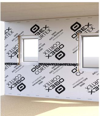
Seal off all edges and joins with OBEX CORTEX 0855 Single-Sided Tape.
