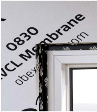
To seal inset corners, cut a section of 0855 Single-Sided Tape and overlay the tape already installed on the inside of the window cutout until any cuts are completely sealed.
