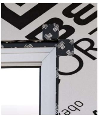
Overlap the previous tape outside of the cutout onto the main area of AVCL to ensure an airtight seal.
