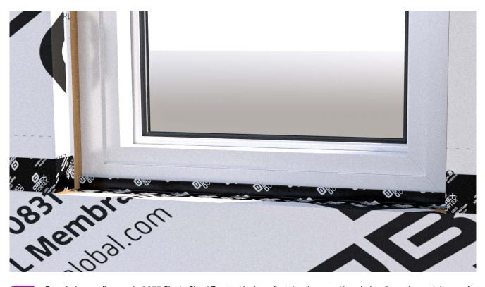
For window sealing, apply 0855 Single-Sided Tape to the base first, lapping onto the window frame by a minimum of 20mm, and ensure adhesion to both the AVCL and the frame.
