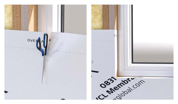
Where possible, the membrane should be continuous so any penetrations should be cut out during application, or it can be applied over the top and cut out afterwards.
