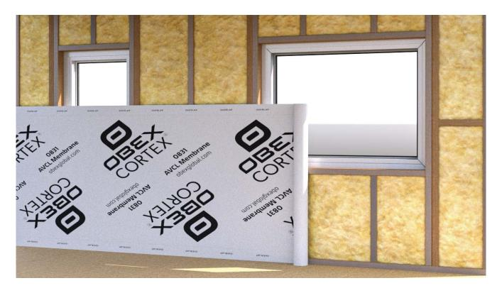
Apply the vapour control layer over the double-sided tape in horizontal strips starting from the base. It is recommended that the next layer should overlap the previous layer by 50mm. The shiny printed layer should be facing into the building (towards the direction of high vapour).
