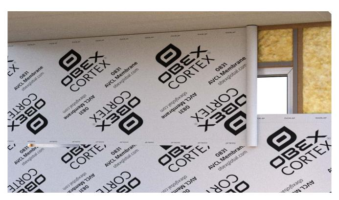
Continue rolling out further layers of AVCL until the section of wall is fully covered.
