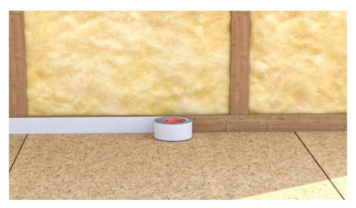
Start by applying the OBEX CORTEX 0850 Double-Sided Tape to the base track. Consider where fixings may penetrate the vapour control layer and ensure that double-sided tape is present at these locations.
