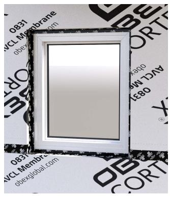
Next seal the sides of the frame, and finally the top edge.
