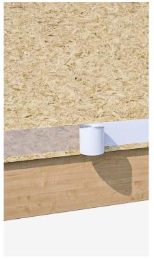
Start by applying the OBEX CORTEX 0850 Double-Sided Tape; 3 strips to cover the width of the membrane (allowance for a 100 mm horizontal lap should be made). Apply tape to ensure all edges of the membrane will be adhered e.g. where the membrane is cut around windows and other penetrations. When you are ready to start installing the breather membrane, peel off the release liner. Some may prefer to remove the release liner as they adhere the membrane.
