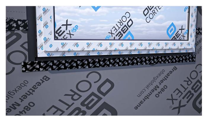
Next seal around the windows starting from the bottom and work upwards. Apply a layer of 0855 to the joint below the window, sealing between the breather membrane and the EPDM.
