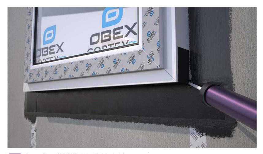
Ensure a small amount of OBEX CORTEX 0769 Paste Adhesive is applied in the corner areas as shown.
