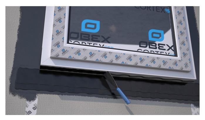
Spread out the 0210FR paste using an adhesive spreader.
