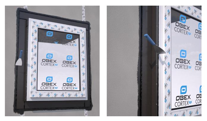
Tool off the paste adhesive using an adhesive spreader and ensure there are no open edges.
