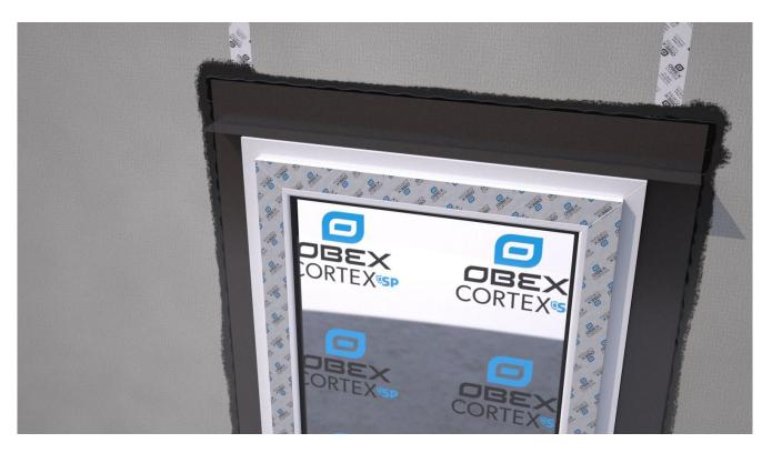
Bond the O200FR Membrane to the frame first, and then bond back to the substrate. Ensure the membrane is applied flat, without creases, and tension free.
