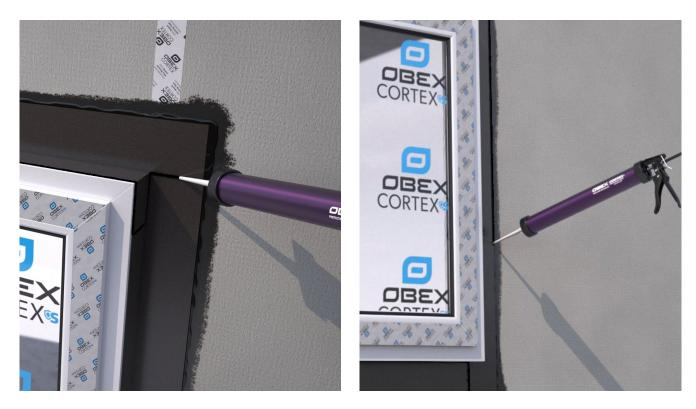
Apply a bead of OBEX CORTEX 0210FR Paste Adhesive around the perimeter and over any joints/overlaps.
