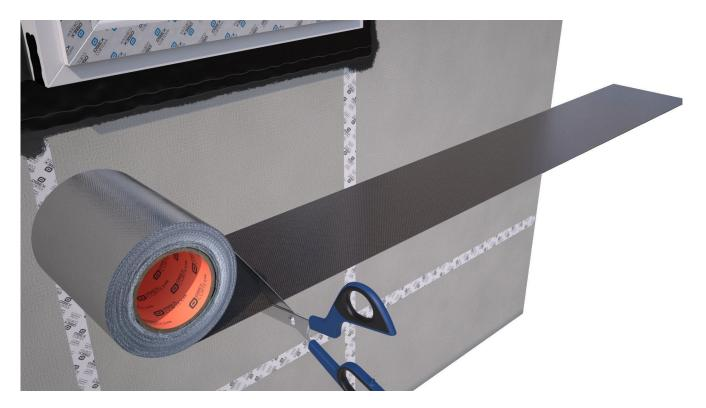
Cut the O2OOFR Membrane to length. Ensure the length of membrane extends at least 100mm past each side of the window.
