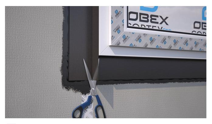
Create an incision as shown by the scissors. Fold and bond the membrane round the frame, ensuring it's applied flat and without creases.
