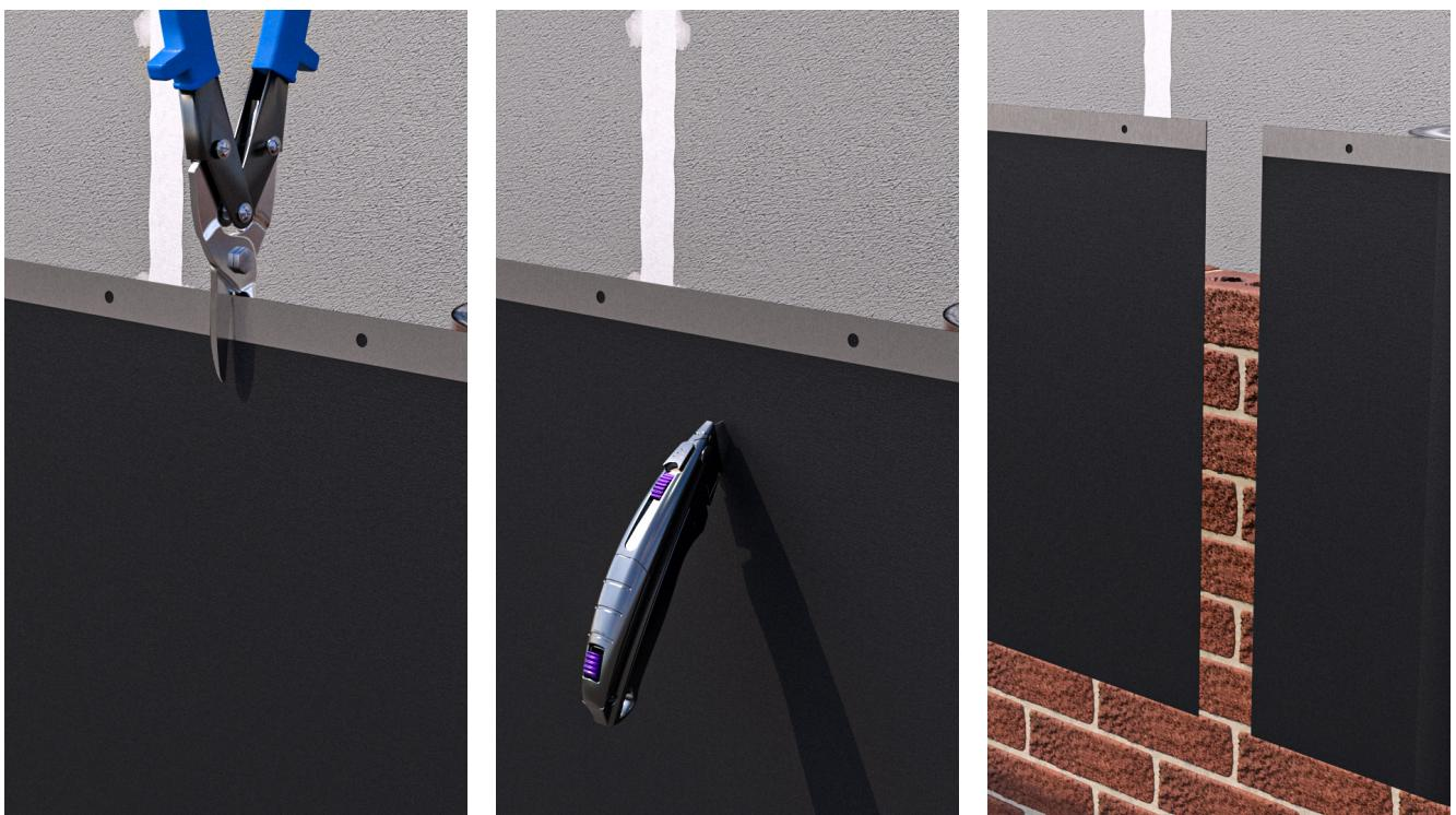
Cut the membrane to length using snips and a knife or membrane shears.
