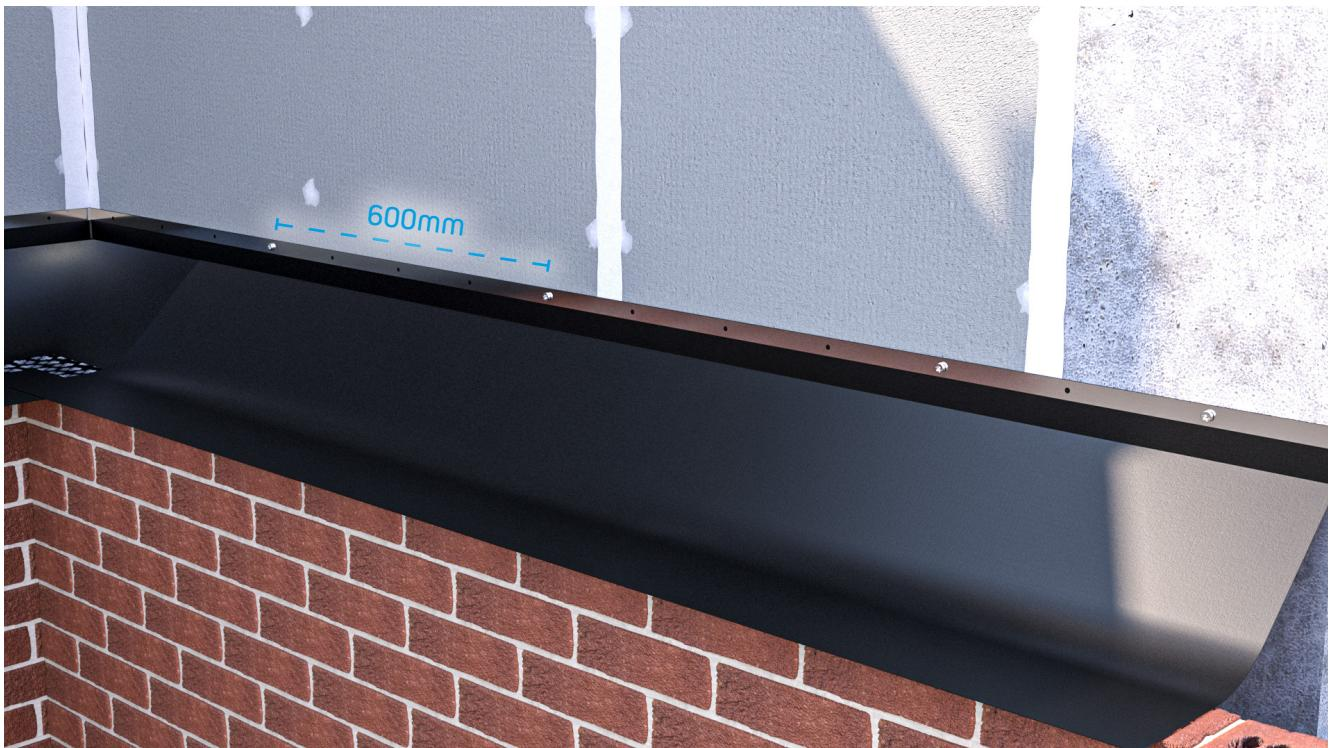
Complete the screws installation, continuing to ensure 600mm maximum spacing between screws.
