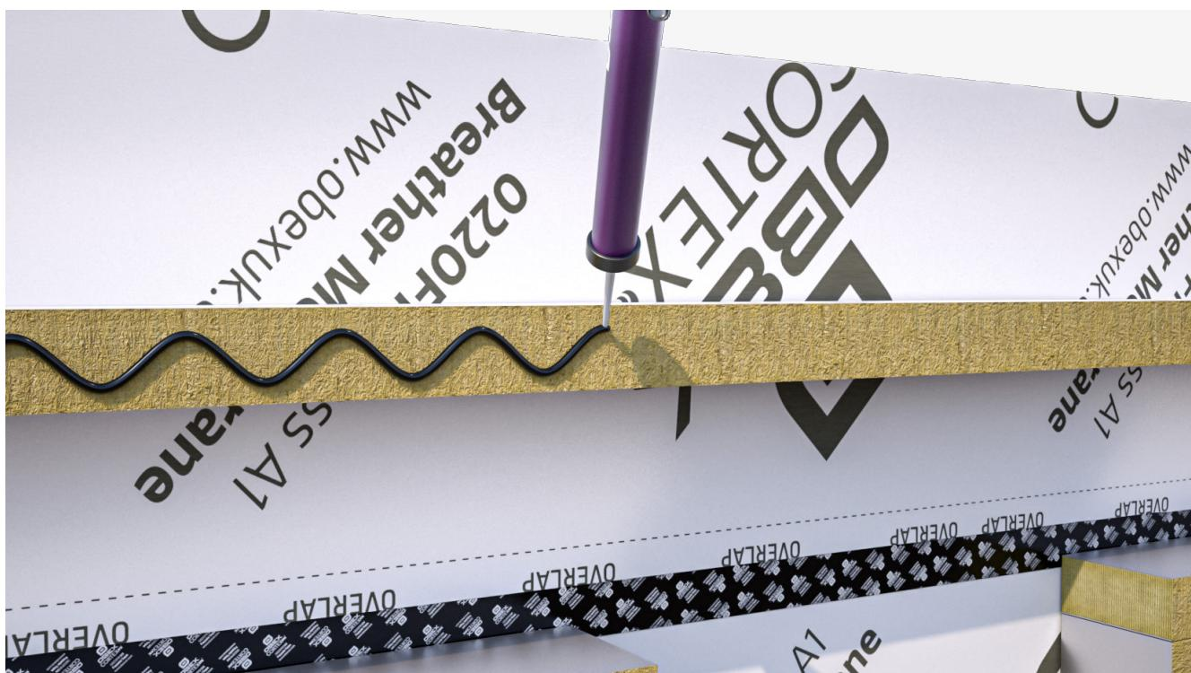
Apply a bead of OBEX CORTEX 0210FR paste adhesive to the outward face of the cavity barrier. Start with the horizontal cavity barriers.
